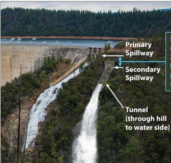
Conceptual rendering of the planned secondary spillway
