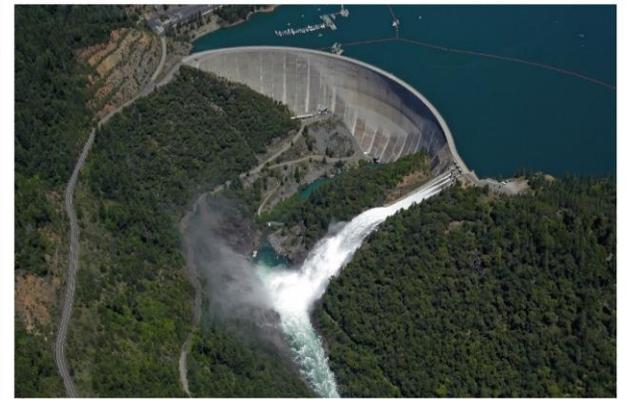
*New Bullards Bar Dam's current spillway releasing water*
